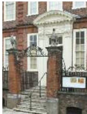
The front entrance of Pallant House
